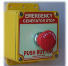
Generator Emergency Stop
